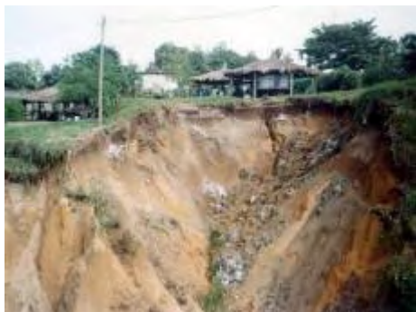
Ravine head threatening public buildings (in DR Congo) Paul Truong, The Vetiver Network, Brisbane, Australia truong@uqconnect.net
