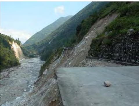
Hailuo沟国家公园道路上的泥石流, Cui Peng , Institute of Mountain Disaster and Environment, Chengdu, China. pengcui@imde.ac.cn
