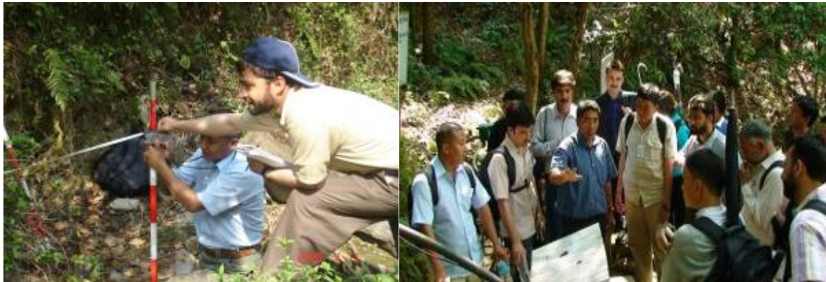
In the photos, field exercise for the check dam construction at the ICIMOD's Demonstration Site, Godavari, Kathmandu, Nepal.
